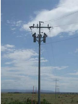
**Aesthetics:** “Our steel poles are uniform in size, and straight with no splinters. Another advantage is that after the steel poles have been installed for awhile, the galvanizing dulls a bit and the poles blend easily into the environment. Our customers notice this and tell us about it,” Cutbirth explains.
