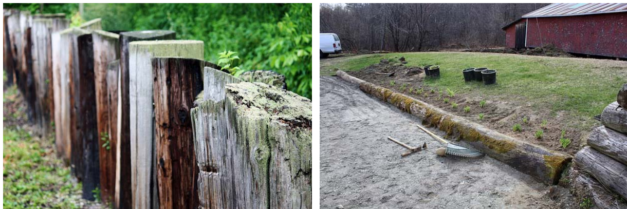
Figure 7. Examples of illegal re-use of treated utility poles, for fence construction in the Southeastern United States. The greenish hue of these poles indicates that CCA was the treatment chemical used. In these situations, these poles represent a severe risk to contamination of local soils from the leaching of arsenic and chromium.
